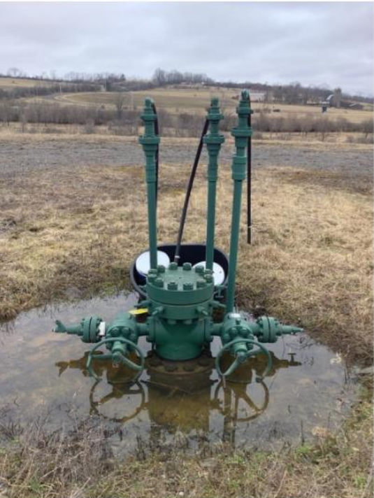
DEP inspection report photo abandoned unconventional well
