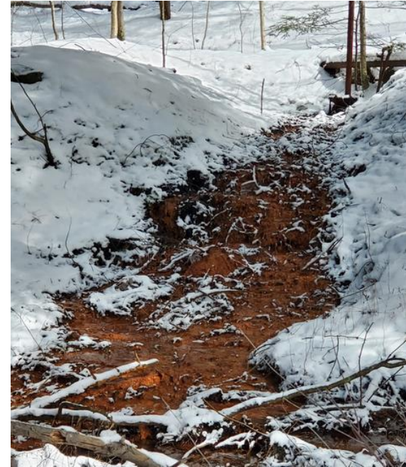
Photo: by Barbara Laxon A leaking plugged well in McKean County 03/21/2024
