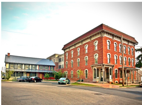
Three Center Square Apartments 2 West High Street, Maytown, PA
