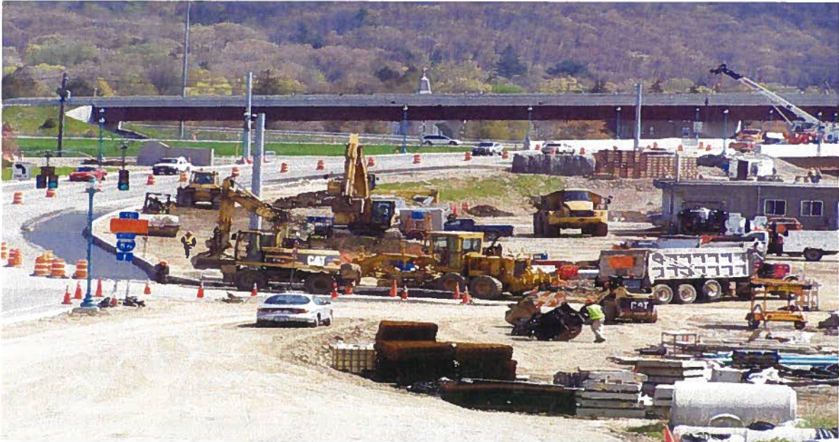
New I-86 / Route 15 Interchange under construction at Painted Post, NY
