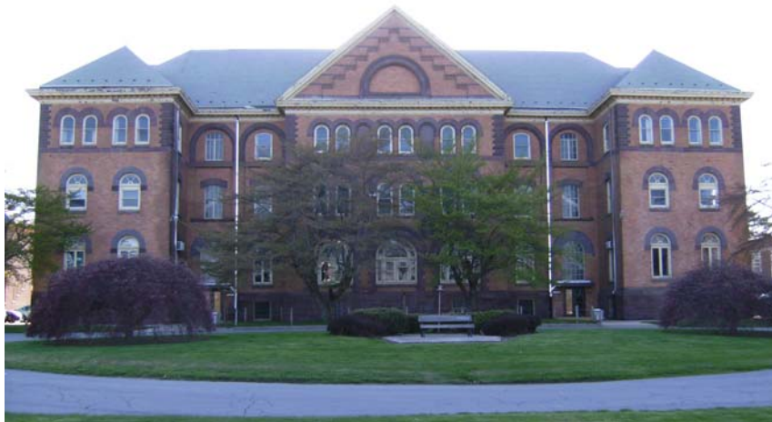
Administration Building SSVC
