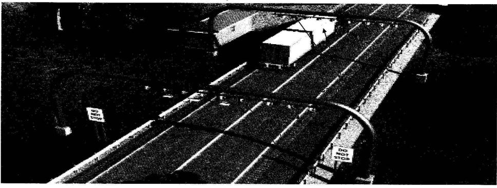
• In the Express "E-ZPass" lanes the front and rear cameras and supplemental lighting are fixed to an overhead the gantry structure across all travel lanes at a height of 19' above the roadway.
