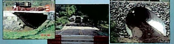
Replace-in-kind, Corrugated Metal Pipe Culverts
