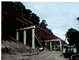
West Kittanning Bridge Armstrong County
