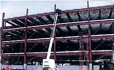
Warren Parking Garage City of Warren
